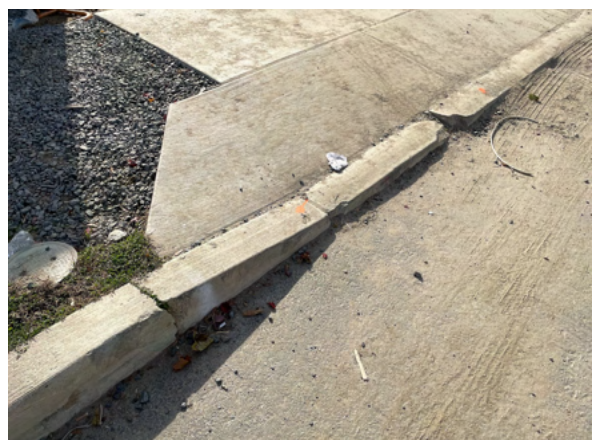
Example of broken concrete at driveway apron
