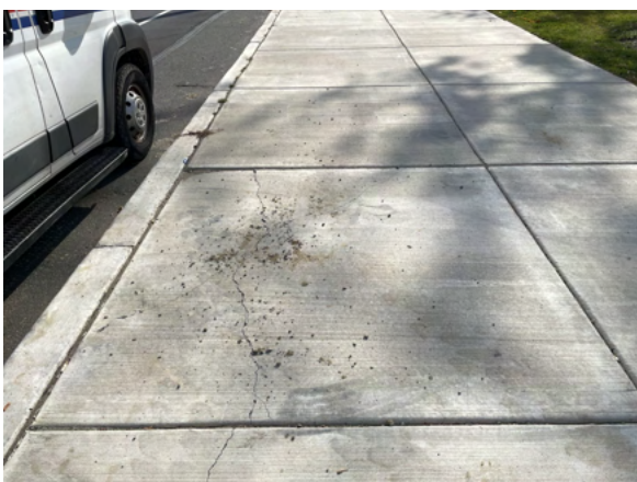
Cracks in concrete - entrance by homesite 1
