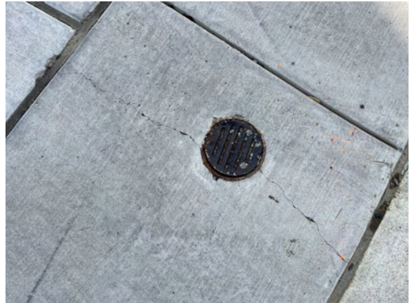
Typical driveway apron sewer vent
