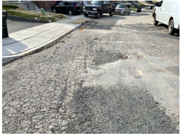
Damage to asphalt base at homesite 15
