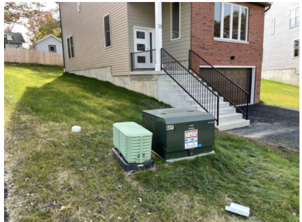
Grading needed at utility boxes
